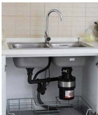
Figure 3. Food waste disposers FWDs (Pictures from the Internet) 图 3. 厨余垃圾处理机(图片来源于网络)
