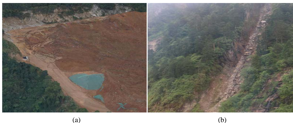
Figure 1. Overview of landslides formed upstream 图 1. 上游形成滑坡概貌
