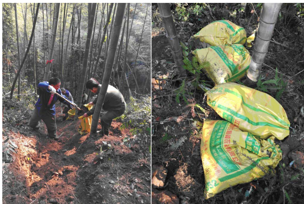
Figure 4. Green exploration trenching 图 4. 绿色勘查槽探施工
