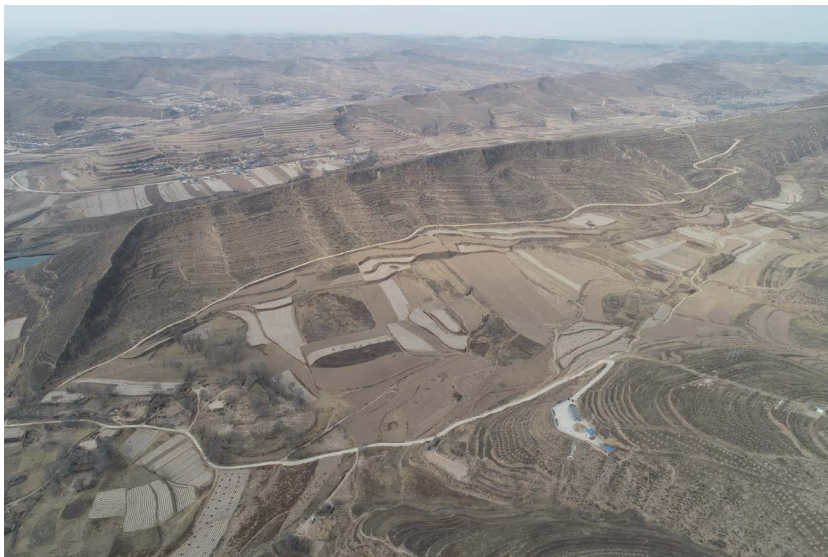
Figure 3. Landslide in Hongtuchuan, Xiji County
