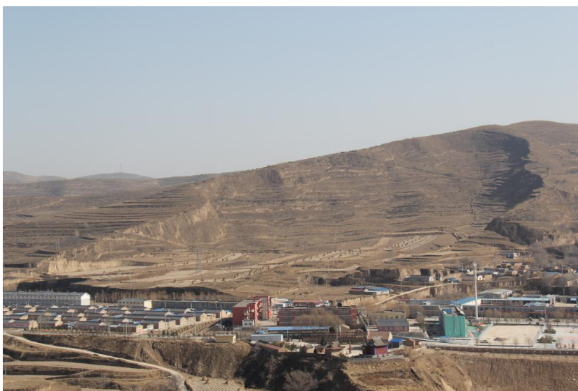
Figure 4. Landslide in Zhenhu Township, Xiji County
