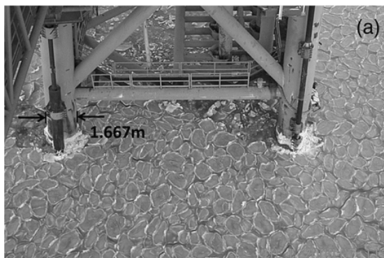
Figure 1. Pancake ice around a jacket platform in Bohai Sea [1]
