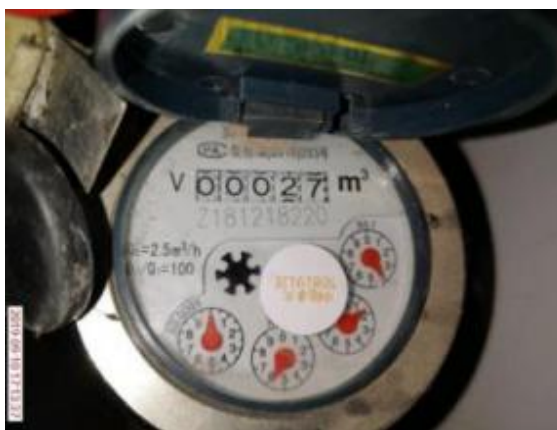
Figure 2. Original water meter image
