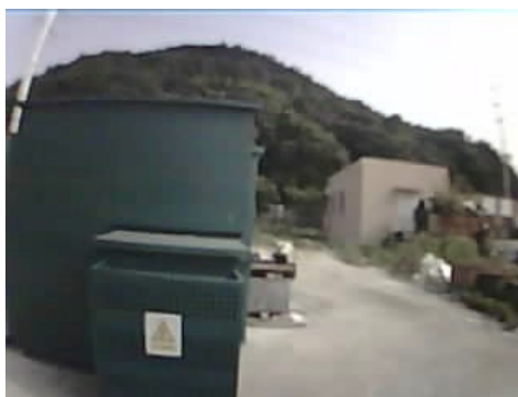
Figure 4. Scenarios of unmanned intrusion into rural power grid substations
