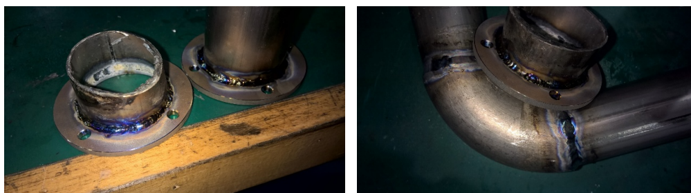
Figure 13. Flange welding completed 图 13. 焊接完成的法兰盘与排气管
