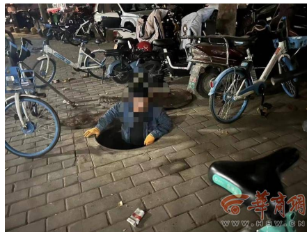
Figure 1. Manhole cover missing 图 1. 人行道井盖丢失 ①
