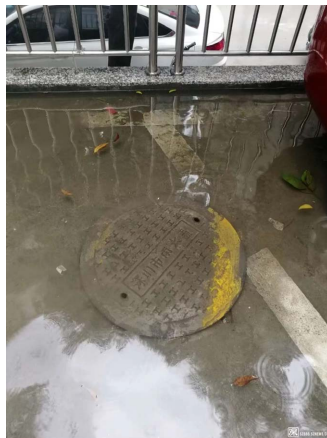
Figure 3. The leaking hole is blocked 图 3. 下水井漏水孔被堵 ③
