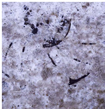
Figure 4. The leaking hole is frozen 图 4. 井盖漏水孔被冰冻 ④
