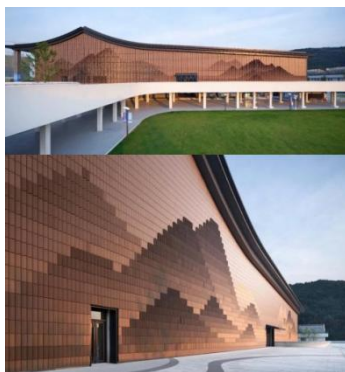
Figure 8. External facade of Fuyang Yinhu Sports Center
