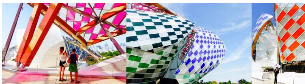
Figure 3. LV foundation building
