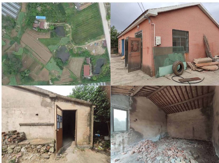
Figure 1. Mengmu homestay in original condition 图 1. 孟墓村民宿原始状态 ①
