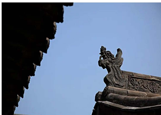
Figure 14. Brick carving decoration on the roof ridge 图 14. 屋脊砖雕装饰 ®
