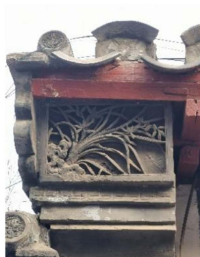
Figure 11. The left steps head of courtyard 137, Lishi Hutong 图 11. 礼士胡同 137 号院左墀头 ®
