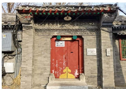
Figure 5. House gate No. 77, east 43
