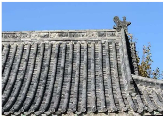
Figure 15. Brick carving decoration on the roof ridge 图 15. 屋脊砖雕装饰 ®
