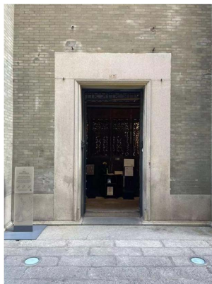
Figure 3. Recessed door 图 3. 凹斗门 ②
