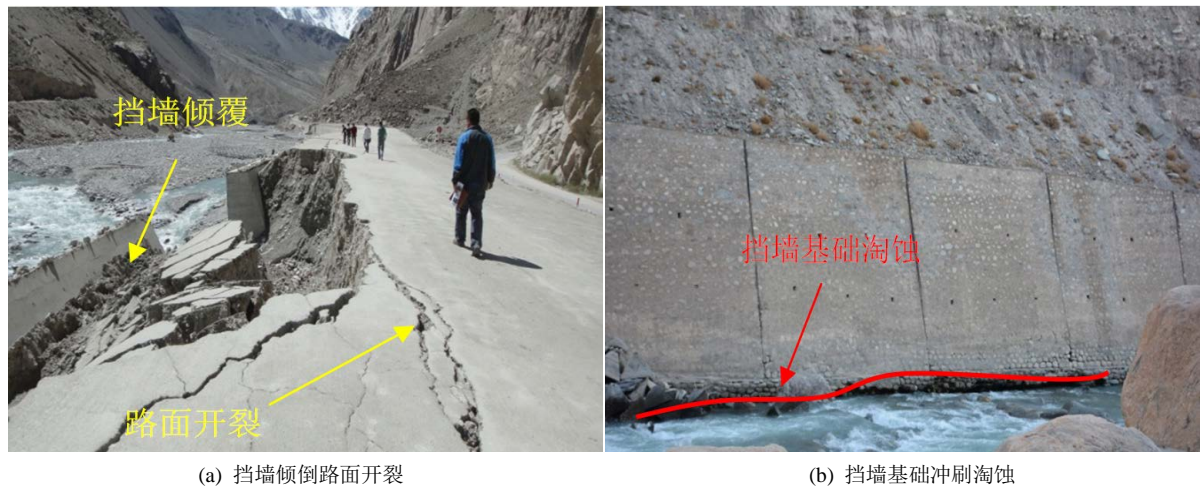
Figure 4. The retaining wall is washed away along the highway 图 4. 公路挡墙冲毁破坏
