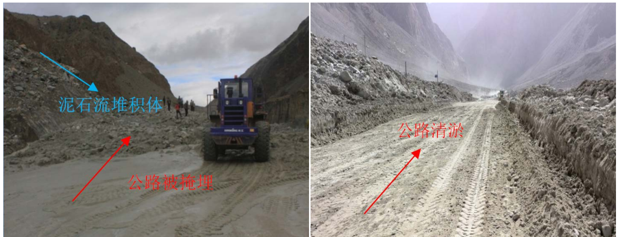
Figure 3. The road in K1600 is buried by debris flow 图 3. 公路 K1600 处泥石流掩埋路面
