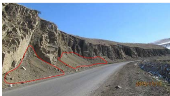
Figure 6. Broken down in K104+760-K104+960 图 6. K104+760-K104+960 段碎落
