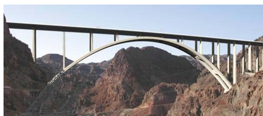
Figure 2. Deck arch bridge composed of two arch ribs and frames 图 2. 双肋框架拱桥 [4]
