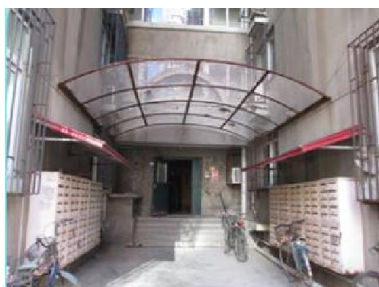
Figure 1. Building entrance of post and telecommunications apartment, Nankai district, Tianjin 图 1. 天津市南开区邮电公寓单元入口
