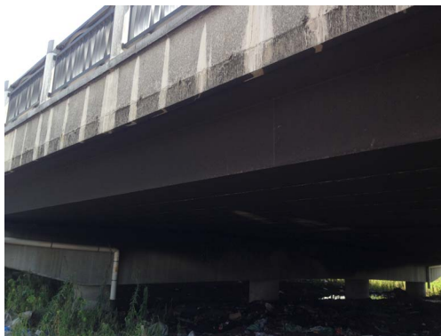
Figure 1. The fired span of bridge 图 1. 受火桥跨
