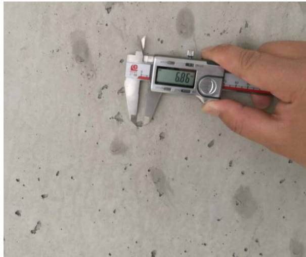
Figure 2. Large bubbles of T-typed beam 图 2. 简支 T 梁大气泡
