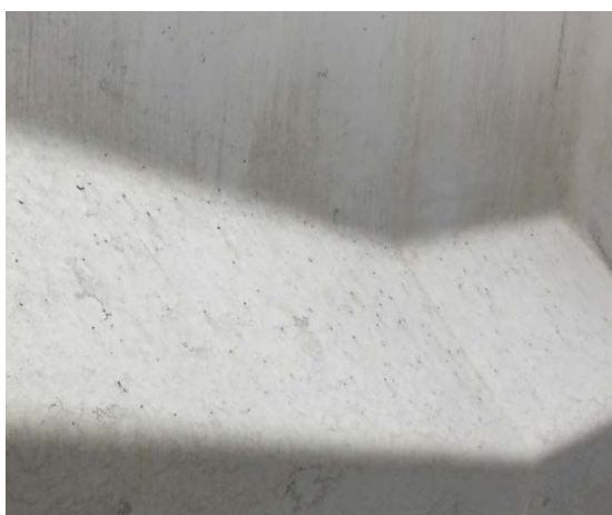
Figure 7. 6# beam's appearance quality
