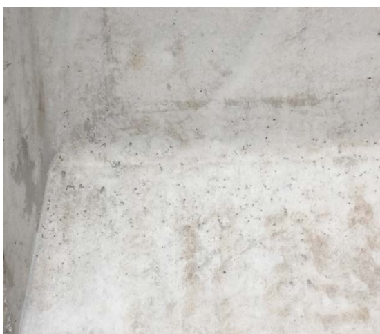
Figure 8. 8# beam's appearance quality
