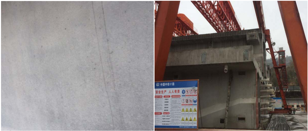
Figure 13. The application effect diagrams in a beam field of Menghua Railway 图 13. 蒙华铁路某梁场应用效果图
