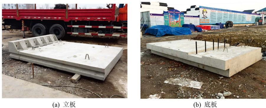
Figure 7. Prefabricated components 图 7. 预制好的构件
