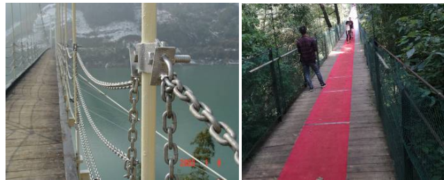
Figure 16. Example of an iron chain and rope flexible railing 图 16. 铁链、绳索柔性栏杆示例
