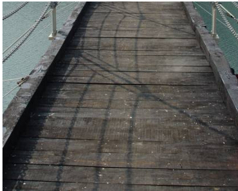
Figure 18. Example of a dispersed bridge deck
