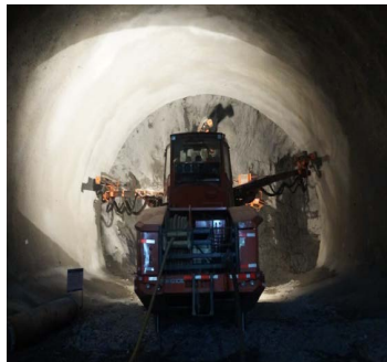
Figure 4. Excavation construction of drilling rig 图 4. 凿岩台车开挖施工
