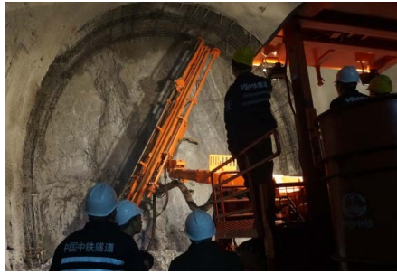
Figure 5. Anchorage construction 图 5. 锚杆施工
