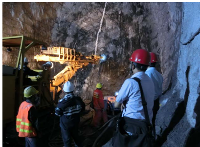
Figure 3. Advanced geological prediction of mine research RPD-180 图 3. 矿研 RPD-180 超前地质预报
