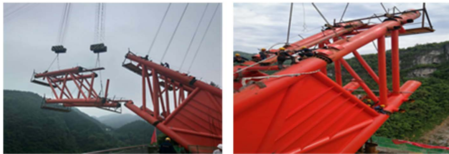
Figure 2. Construction drawing of zhaolongba bridge section hoisting 图 2. 找龙坝桥节段吊装施工图
