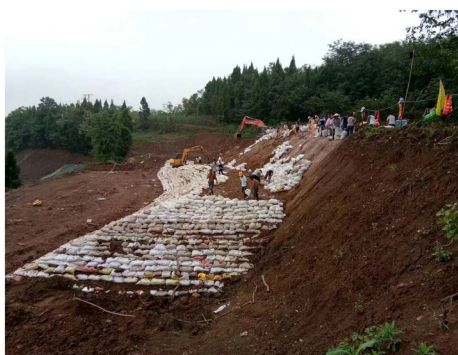
Figure 5. Ballast in front of the landslide 图 5. 滑坡前缘压脚
