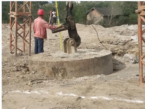
Figure 5. The measurement of the settlement 图 5. 夯沉量测量
