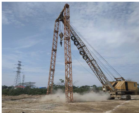
Figure 4. The test of the first construction 图 4. 试夯
