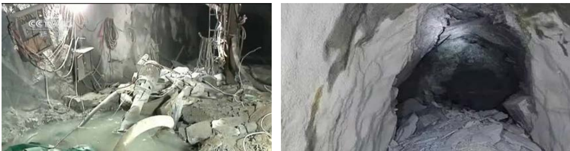
Figure 1. The phenomena of rock burst
