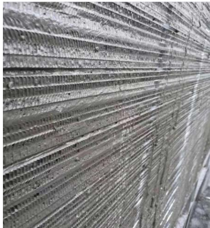
Figure 3. Back wall of concrete building 图 3. 混凝土建筑后墙身
