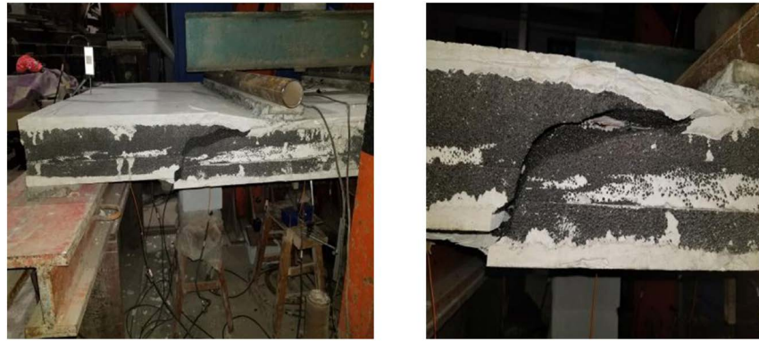
Figure 12. Detail of specimen destruction 图 12. 试件破坏细部图
