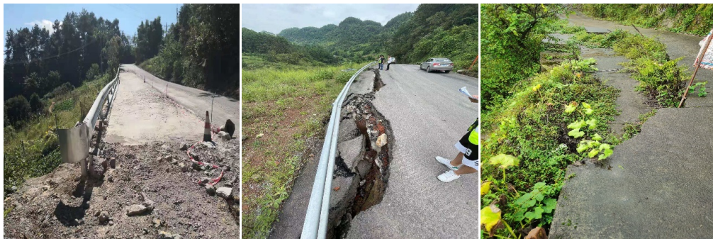
Figure 3. Investigation map of subsidence and collapse site 图 3. 沉陷塌陷现场调研图
