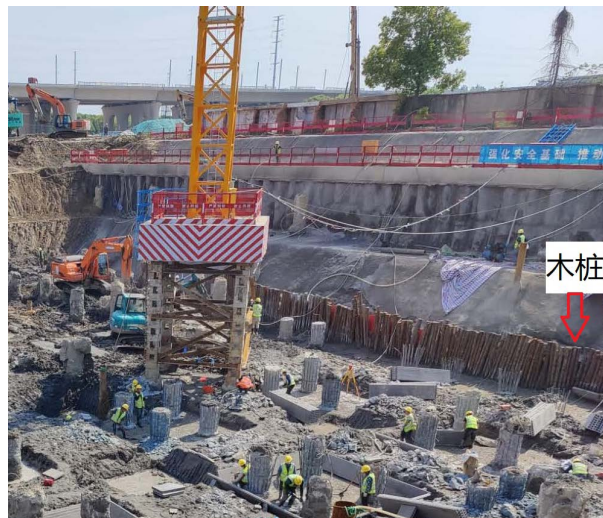
Figure 9. Photo of site excavation after consolidation with timber piles
