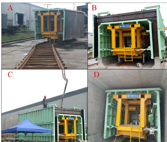
Figure 14. Engineering test of working performance of hydraulic formwork trolley 图 14. 液压模板台车工作性能的工程试验
