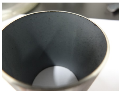
Figure 3. High temperature reheater tube 图 3. 高温再热器管
