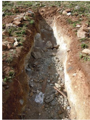
Figure 1. Test pit of in situ direct shear 图 1. 原位直剪试验坑槽
