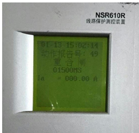
Figure 3. Line reclosing protection action diagram 图 3. 矢崎线重合闸保护动作图
