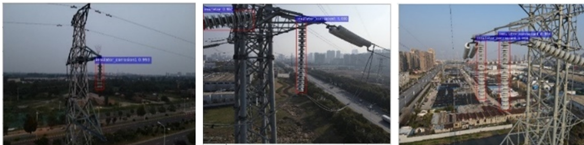
Figure 2. Detection results of insulator strings in visible images 图2. 可见光图像中绝缘子串的检测结果
