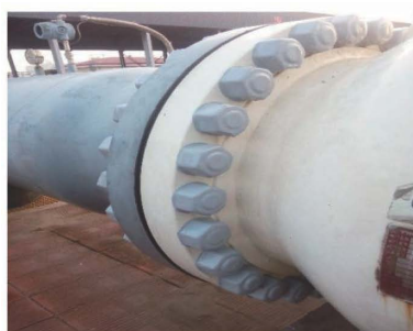
(a) 输油站阀体螺栓防腐修复
