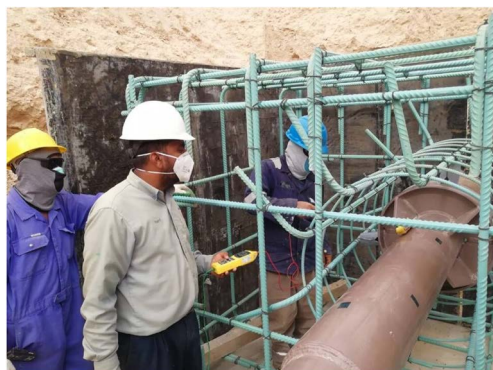
Figure 14. Holiday inspection 图 14. 防腐层检漏
