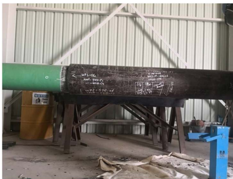
Figure 6. Welding of sleeve
