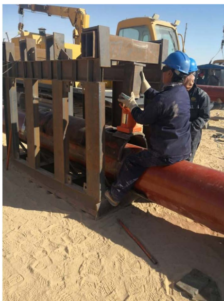
Figure 5. Squeeze of sleeve
