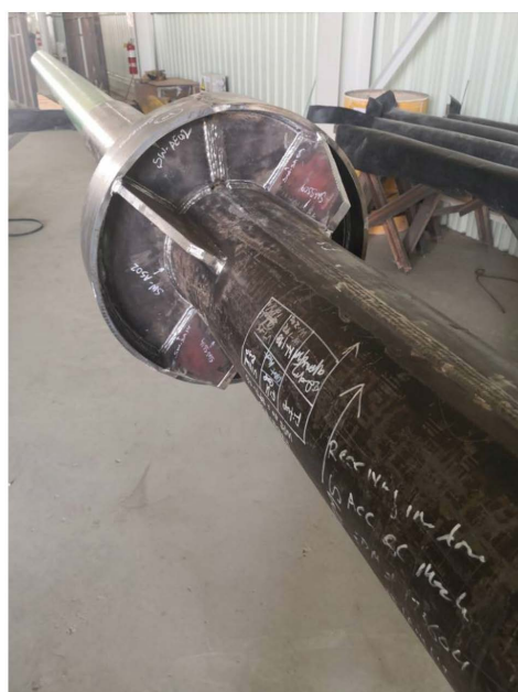
Figure 7. Welding of stiffener plate
