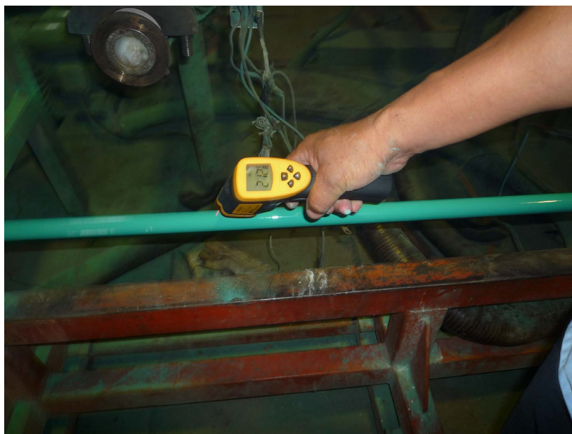
Figure 2. Temperature inspection after spraying 图 2. 喷涂后温度检测
