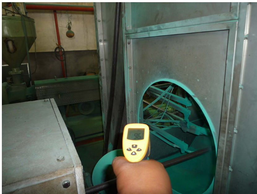
Figure 1. Temperature inspection before spraying 图 1. 喷涂前温度检测
