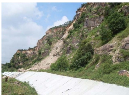
Figure 1. Typical excavation slope status in the second section
