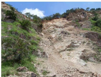
Figure 2. Status of collapse and destruction of the second section
