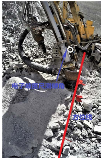
Figure 2. On-site measurement and control construction 图 2. 现场测控施工
