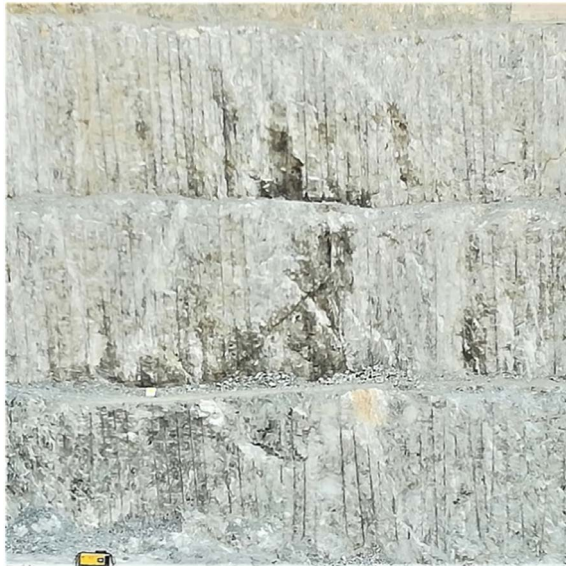
Figure 3. Half-wall hole of pre-split hole
