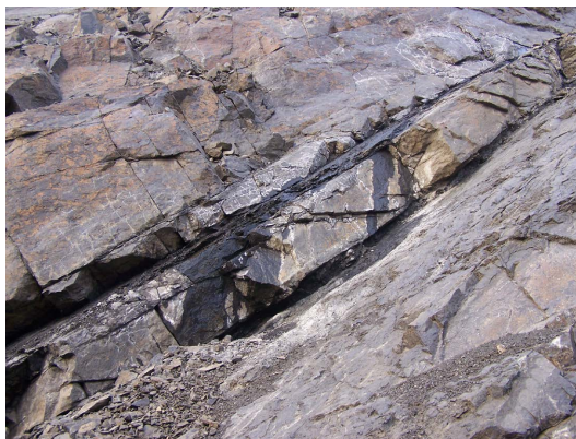
Figure 1. Landslide failure of bench slope 图 1. 台阶破滑坡破坏
