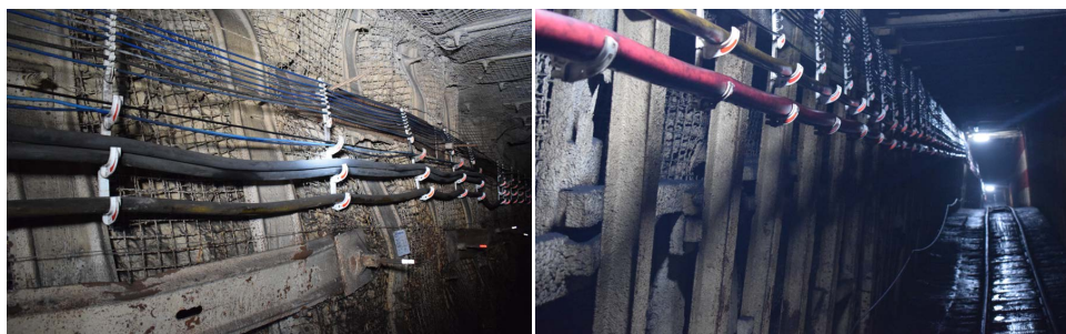
Figure 8. Schematic diagram of air leakage channel blocking along the air side 图 8. 沿空侧漏风通道封堵示意图
