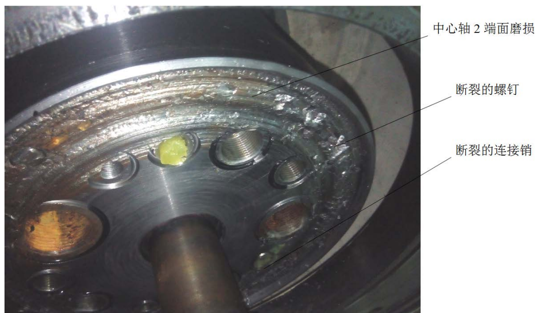
Figure 2. Fracture of bolt and pin in C-C section
