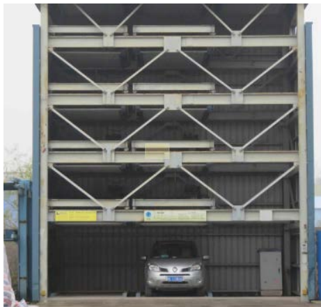
Figure 1. Lifting horizontal moving intelligent garage 图 1. 升降横移式智能车库
