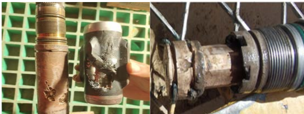
Figure 3. Damage caused by erosion and blocking jams 图 3. 冲蚀、阻卡造成的损坏情况
