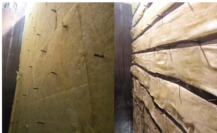
Figure 2. Working sketch of the flexible felt at the test site 图 2. 试验现场弹性毡施工效果图
