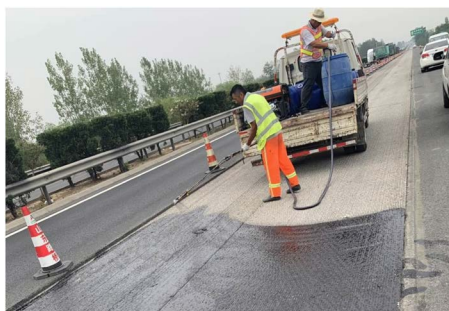
Figure 6. Spraying high performance trackless emulsified asphalt 图 6. 高性能不粘轮乳化沥青喷洒
