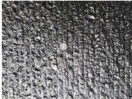
Figure 4. Spraying high performance trackless emulsified asphalt on milling surface 图 4. 铣刨面上喷洒高性能不粘轮乳化沥青
