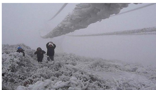
Figure 1. Zhaotong transmission line icing ( >20 mm)
