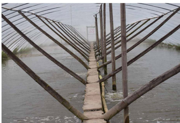
Figure 1. Internal structure diagram of Rudong shed culture mode 图1. 如东小棚养殖模式内部结构图
