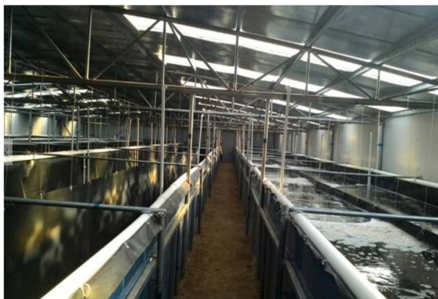
Figure 3. Internal structure diagram of Rudong shack in recirculating aquaculture 图 3. 循环水养殖如东小棚内部结构示意图
